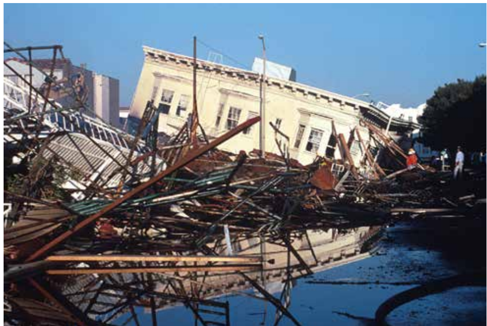
The result of an earthquake
